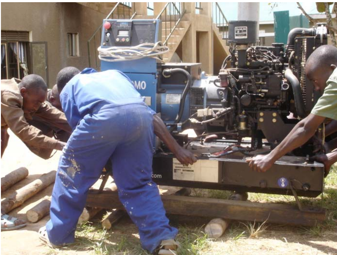
Moving one of the generators
