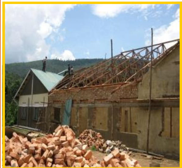
Doubling capacity of the Maternal Health unit: work in progress.
