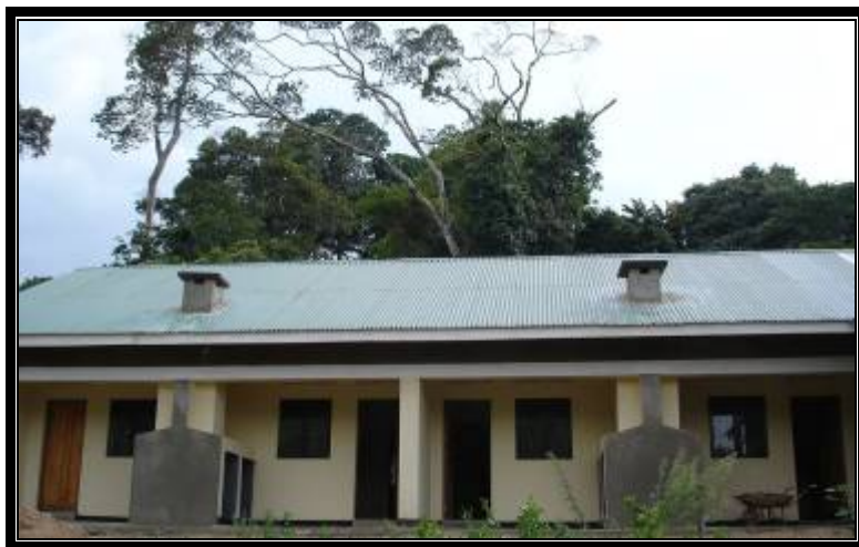
Some of the new staff housing units with power and water – the accommodation committee chose the lucky recipients
