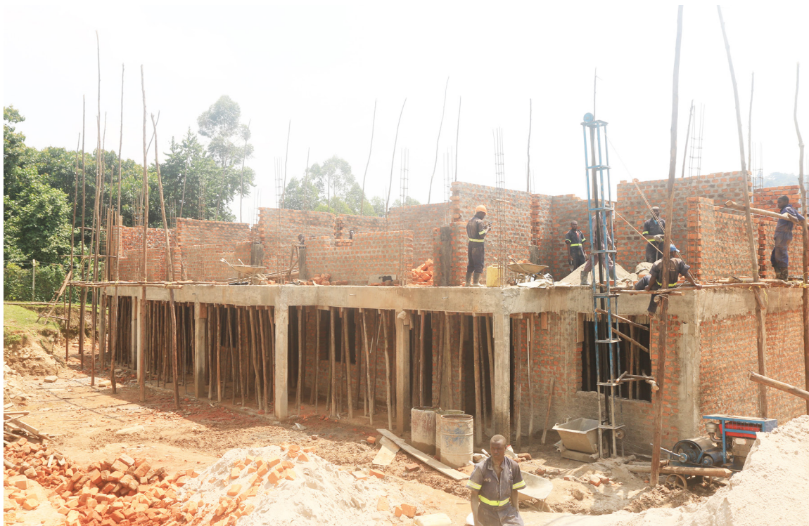
Midwives accomodation facility under construction.
