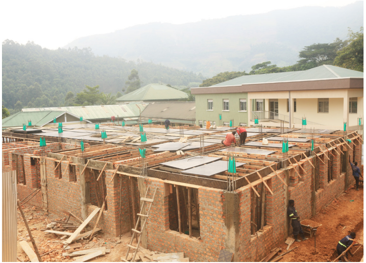
Medical ward that will house Intensive Care Unit under construction
