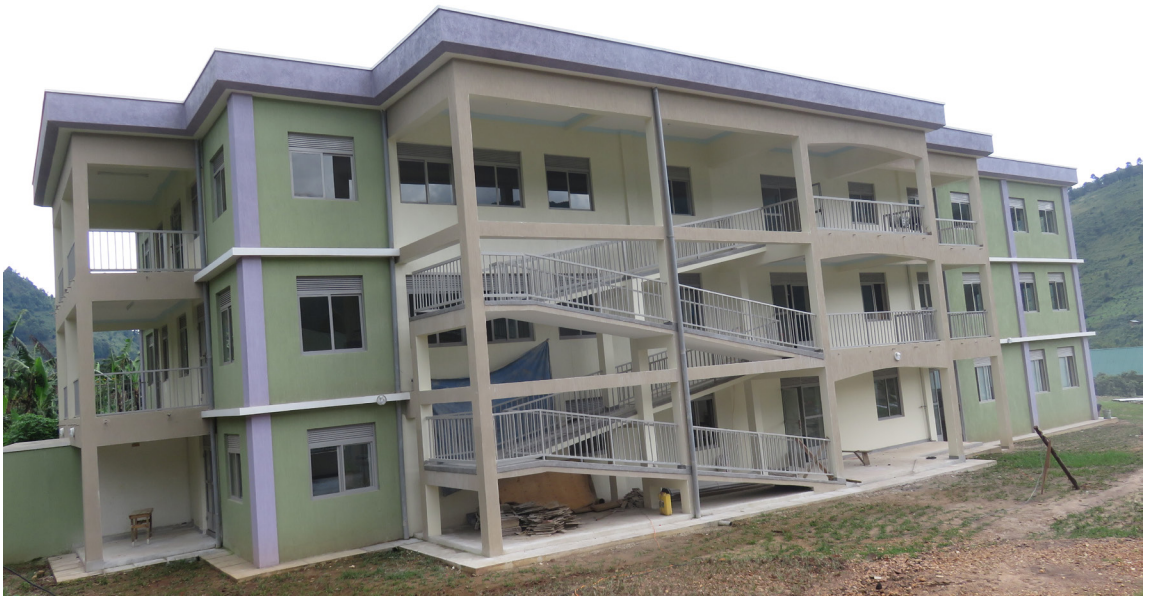
The new skills laboratory/ library at the nursing school
