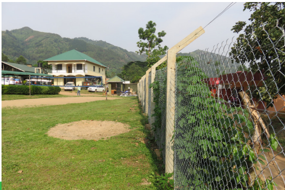
The new Hospital Fence
